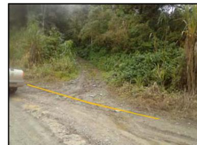
1+625 a 1+635 - LD - Executar travessia com tubo de Ø60; Comprimento = 10,00m;
